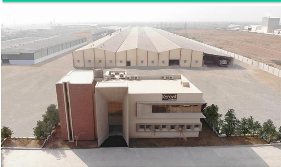
Sanitaryware 1 st Plant, Gujarat
