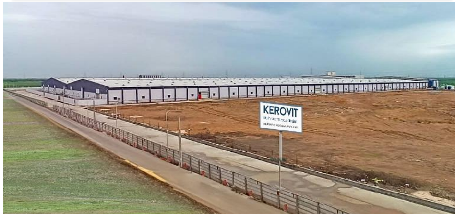
Sanitaryware 2 nd Plant, Gujarat
