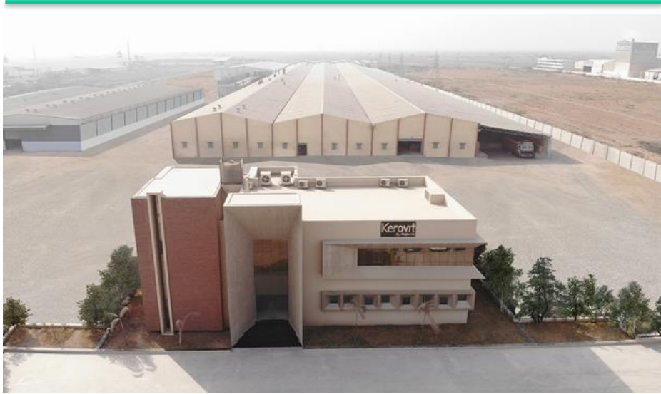
Sanitaryware 1 st Plant, Gujarat
