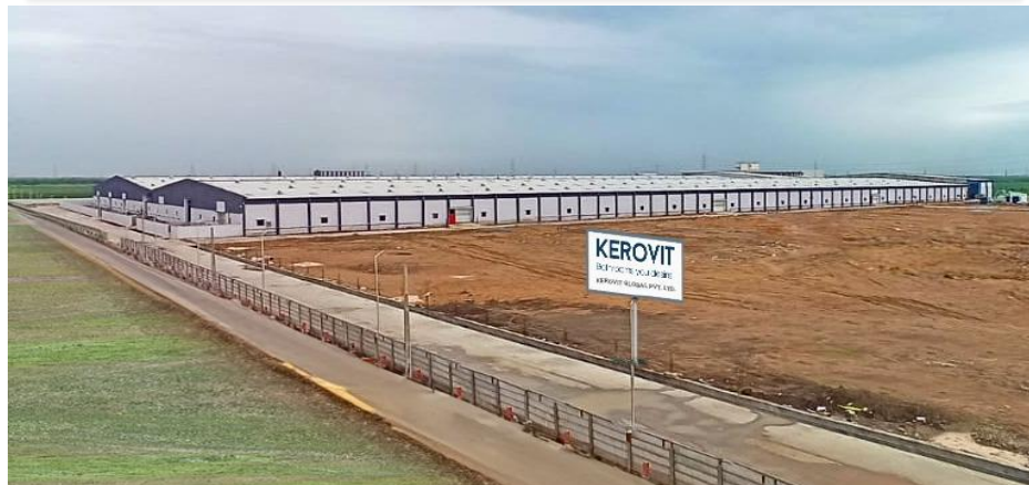
Sanitaryware 2 nd Plant, Gujarat
